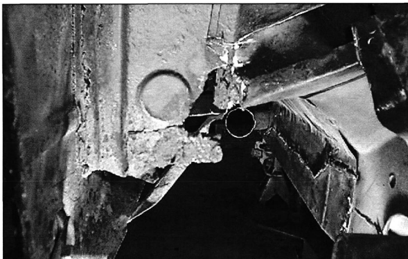
This is a rear view before the “hole” was created.
