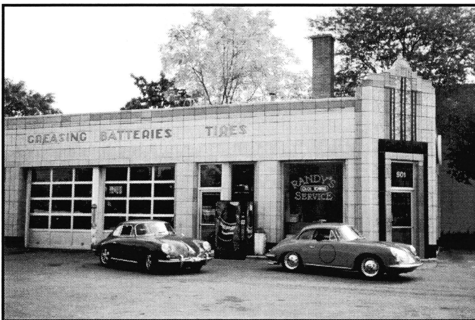
The Skirmants' and the Downey's stop for a great "vintage look" photo opportunity at Randy's Service in Traverse City
